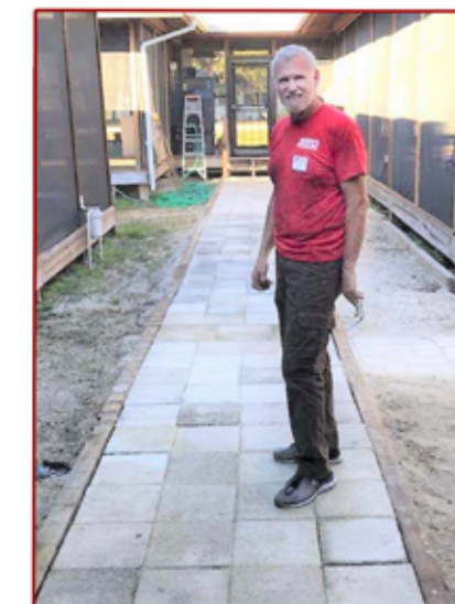
One Walkway Completed
