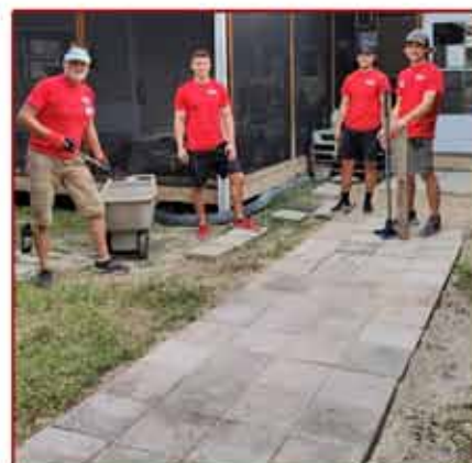
Creating a New Brick Walkway
